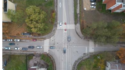
Figure 5. Crossing in Location 3
